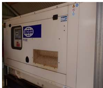
Figure 3-2 Diesel Generator at Water Treatment Plant, rated at 110kVA [photo: Enhar]
