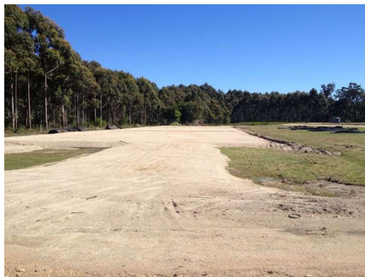
Figure 6-44: Foundation for kitchen to compost area adjacent to sewage treatment works [photo by Enhar, November 2013]
