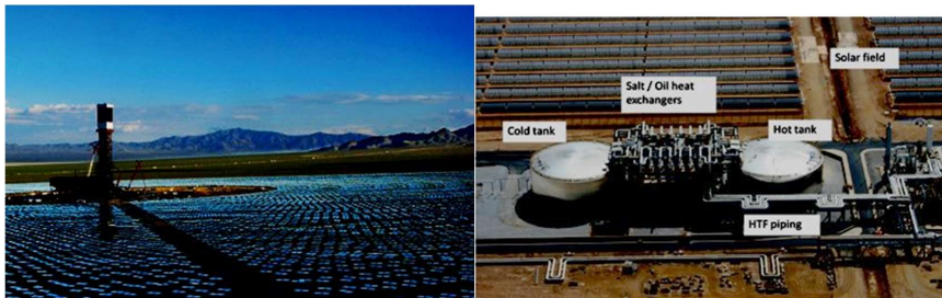
Figure 6-23 [Left] Ivanpah CST Power Station (Source: Ivanpahsolar.com) [Right] Molten Salt Thermal Storage System (Source IT Power 2012)
