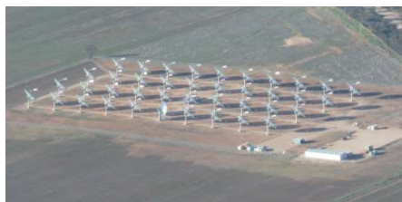
Figure 6-14-1, 1.5 MW Concentrated Photovoltaic demonstration facility in Mildura.
