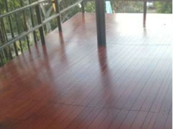
HARDWOOD FLOOR DECKING - NO GAPS - BAL40/FZ RATING
